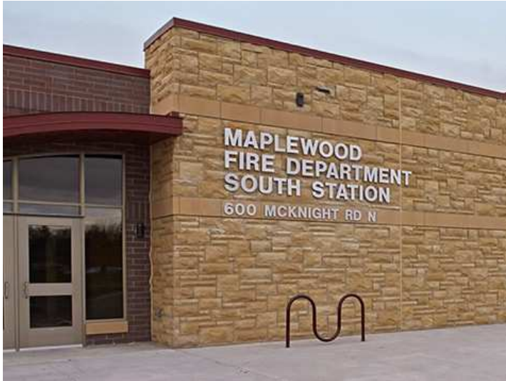
Maplewood South Station Fire Department
