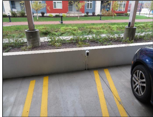
Future Level 2 EV charging station at Galloway Ramp Eau Claire, WI 2019 (City of Eau Claire)
