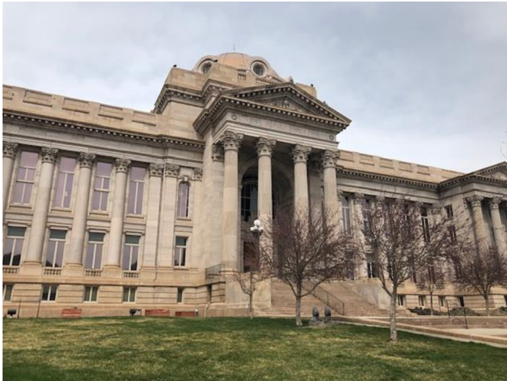
Figure 4: Pueblo County Court House, Photo Credit: Brendle Group
