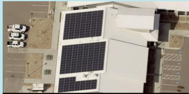
Modeled Solar Panels on Town Public Services Facility
