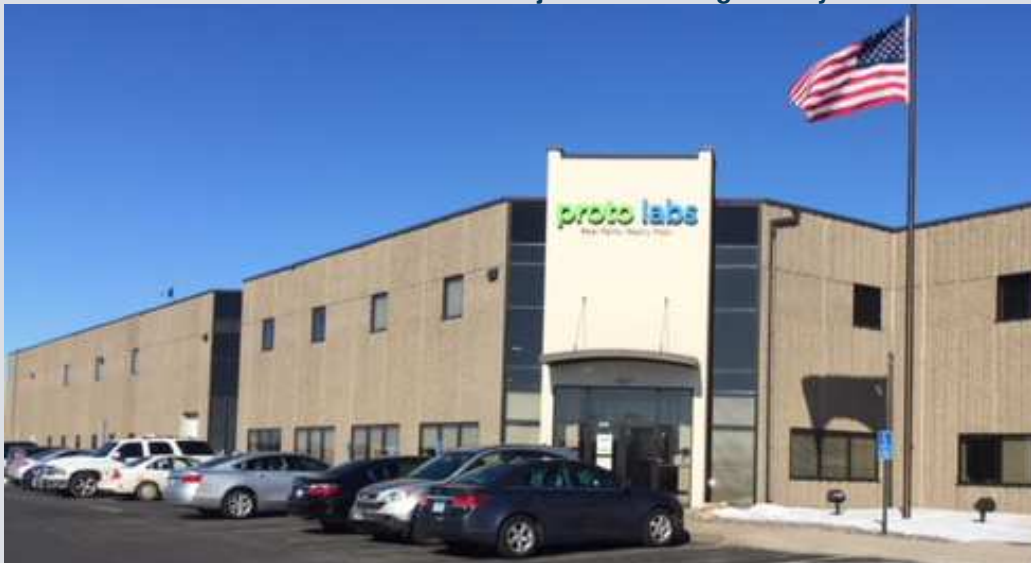
Proto Labs Rosemount Injection Molding Facility
